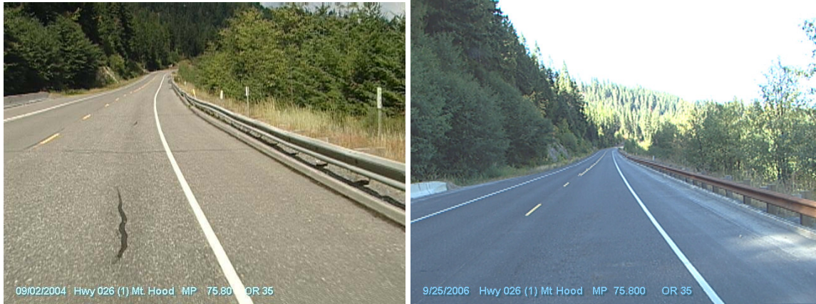
Figure 5.36: Conditions in 2004 (before) and in 2006 (after) showing the preservation work at MP 75.80
