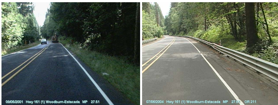
Figure 5.30: Conditions in 2001 (before) and in 2004 (after) showing the added guardrail/upgraded culvert at Little Cedar Creek (MP 27.51)
