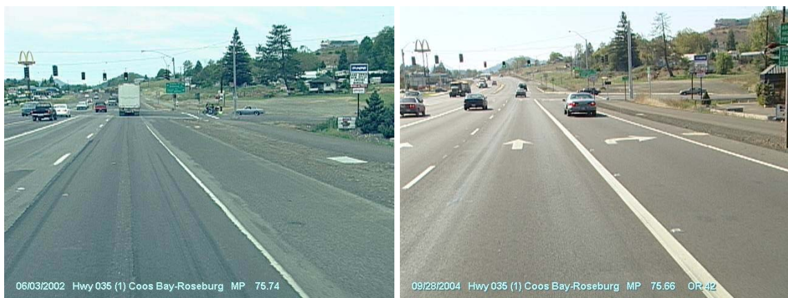
Figure 5.4: Conditions in 2002 (before) and in 2004 (after) showing the addition of the right-turn lane at “Kelly’s Corner” MP 75.72. OR-99 improvements not shown.
