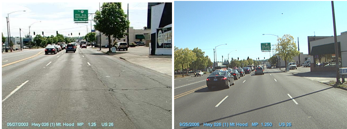
Figure 5.19: Conditions in 2003 (before) and in 2006 (after) (2006) showing the overlay at MP 1.25
