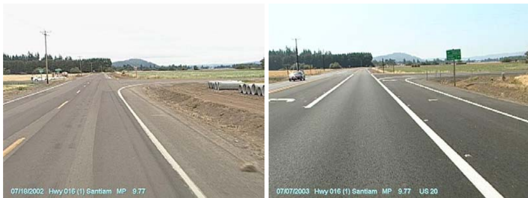
Figure 5.2: Conditions at Spicer Rd in 2002 (before) and added turn lanes in 2003 (after)
