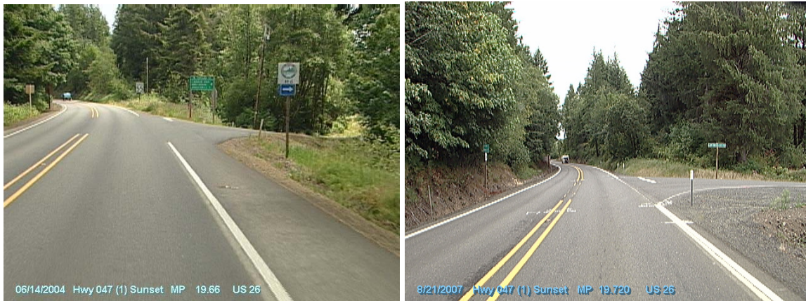
Figure 5.49: Conditions in 2004 and in 2007 (after) showing the Nehalem Road realignment at MP 19.72
