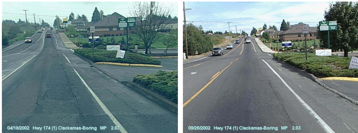
Figure 5.10: Conditions in 2001 (before) and 2002 (after) showing the preservation work at MP 4.93 and the area near Royer Road (no median installed)
