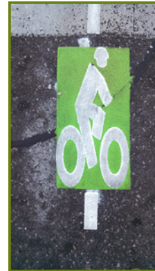
Installed “Green Backed” Stencil
