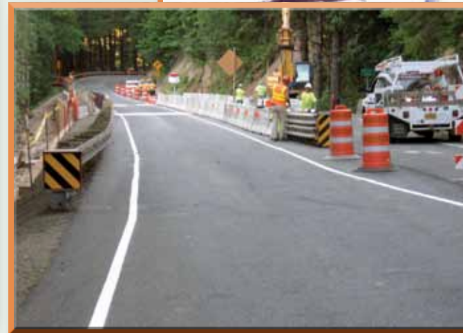
An undersized culvert on the Umpqua National Forest's Williams Creek hindered both aquatic and terrestrial passage across the highway. Umpqua National Forest staff worked hard to obtain funding, including funding from the American Reinvestment and Recovery Act, to replace the culvert with a bridge that will enable aquatic and terrestrial passage when completed. (Images: USDA Forest Service)
