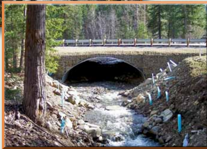
Replacing culverts to enable aquatic passage does not always help to increase wildlife passage, but it did in this example on Little Boulder Creek in Washington. Perched culverts are barriers to many terrestrial wildlife species as well as aquatics. A wider opening combined with natural substrate of small to moderately sized materials facilitates passage by many terrestrial animals. (Images: Washington DOT)
