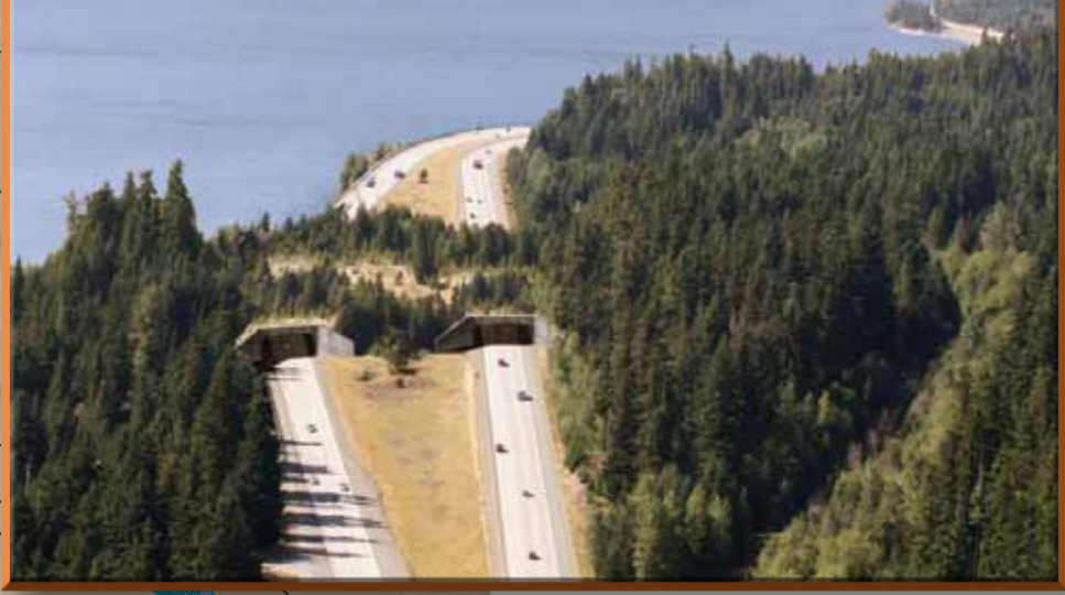
Overpasses covered with vegetation are a tiny ecosystem of connectivity across the heavy traffic and several lanes of an interstate highway. When built as part of the Snoqualmie Pass project, the Noble Creek wildlife overcrossing will help restore habitat connectivity for wildlife and plants across Interstate 90. Huge, complex projects such as this take years to plan and a great deal of dedicated staff time from resource agency personnel as well as the DOTs. (Simulated Image: Washington DOT)
