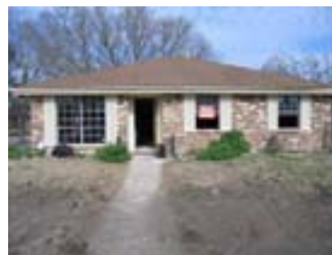
house on slab foundation
