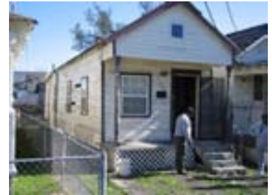
house on pier foundation
