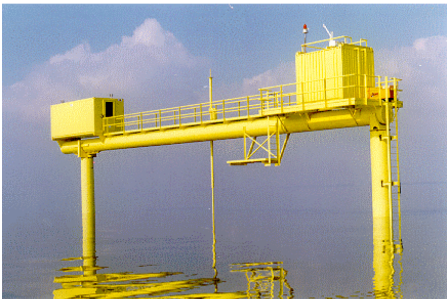
Figure 4.1 Picture of the BOA bridge
