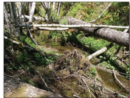
B —Felled alders and newly placed wood worked together to catch coarse woody debris coming downstream and improved channel functions and complexity almost immediately.
