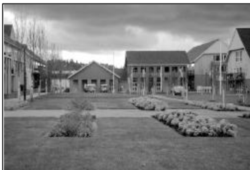
Phase I of Russellville Commons contains 282 units of market rate housing with interior green space and community amenities
