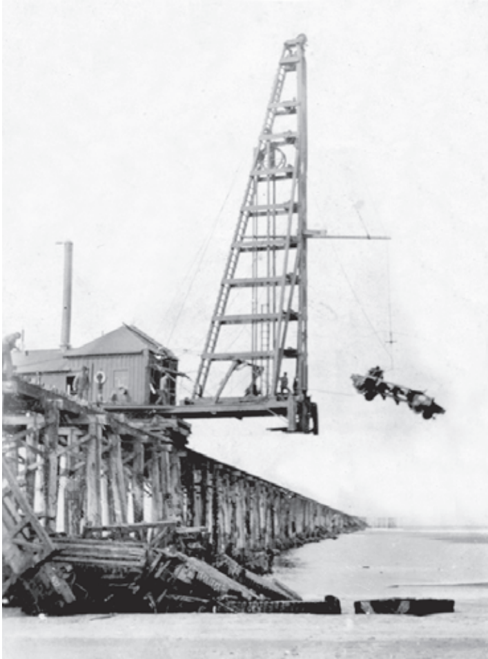
Figure 9.12 – The construction of falsework trestles on the north jetty, adjacent to the base of Cape Disappointment, in the 1910s. Photo courtesy Washington State Historical Society.
