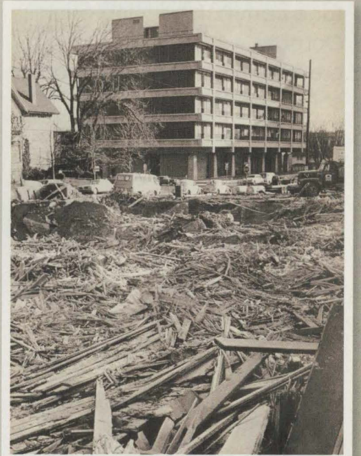
A group of enterprising students, including Stan Amy (top), saved buildings marked for demolition, and managed them as student housing. Photos from the 1969 Viking Yearbook.
