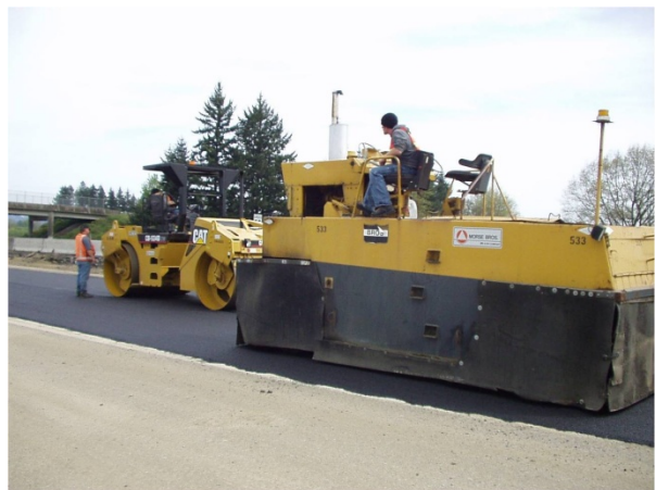
f) Compacting second lift of HMA.
