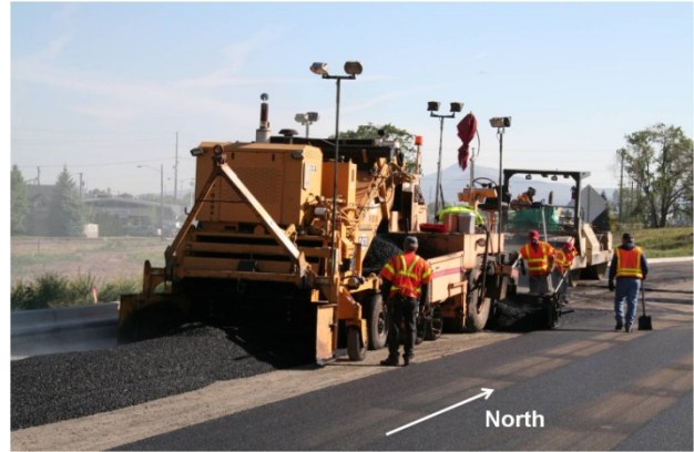
b) Windrow elevator attached to paver.
