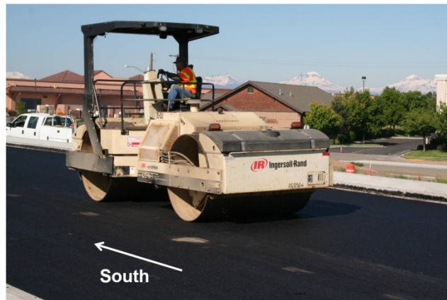
c) Compacting the first lift of HMA with a heavy roller.
