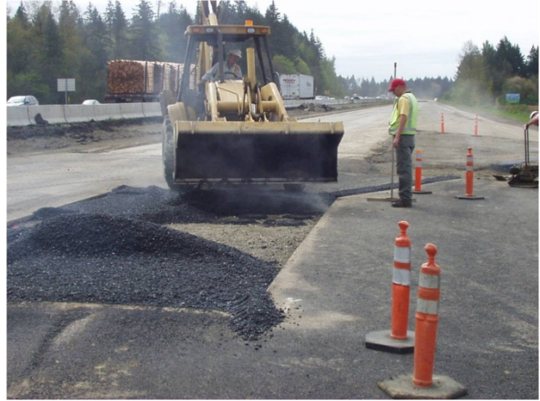
b) Covering gages with HMA.
