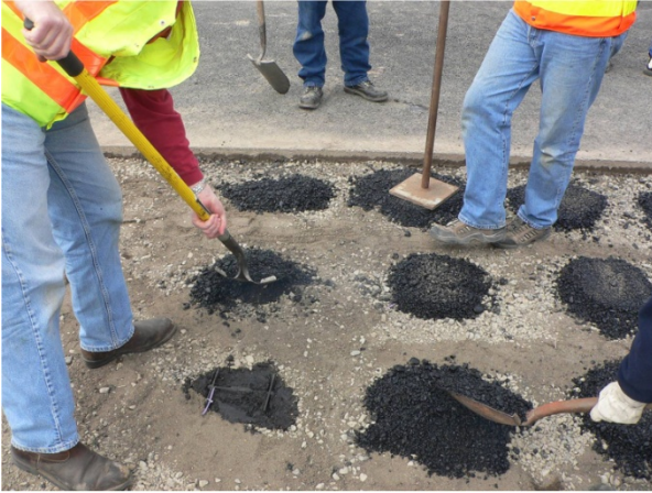
a) Protecting gages with loose HMA.
