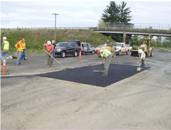
c) Spreading HMA over gages.
