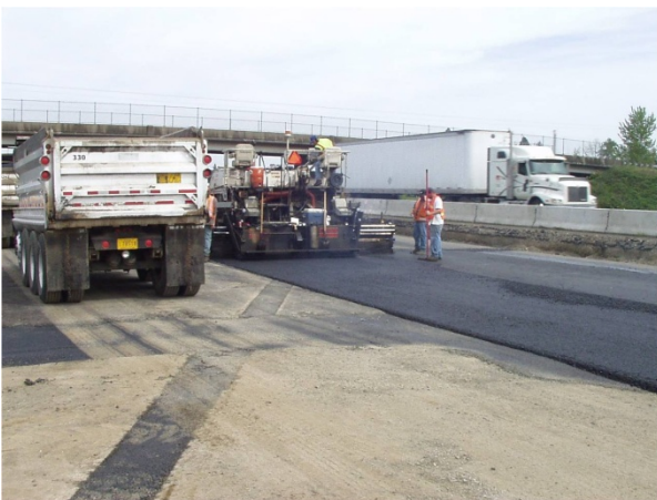
e) Paving second lift of HMA.
