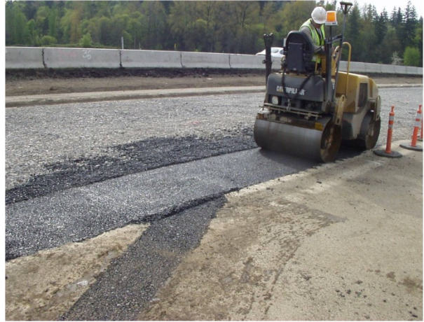
b) Compacting HMA with a small roller.
