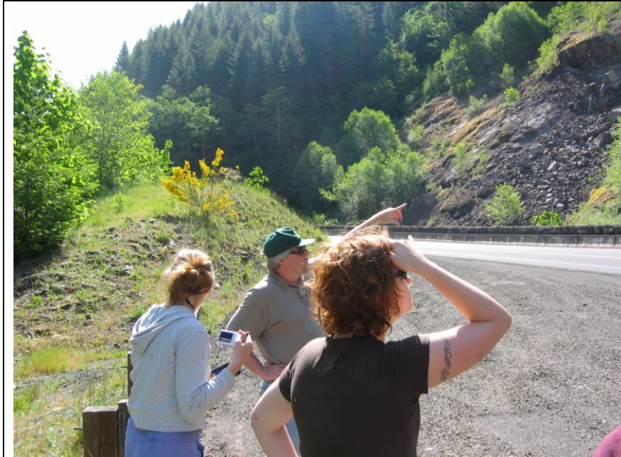
Keith Mills, ODF, pointing out landslide on Highway 8 caused by road construction at top of slope.
