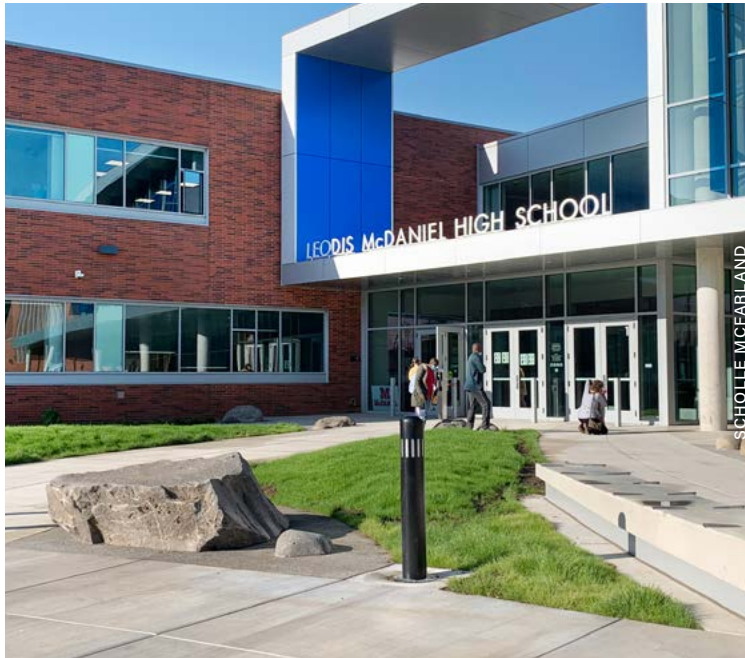
The newly renovated Northeast Portland school once known as Madison High reopened this September with a new name that pays homage to past principal Leodis V. McDaniel.
