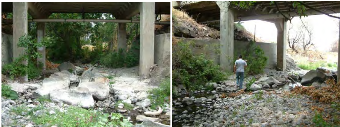
Figure 4.12: Site 10 - Chenoweth Creek downstream and upstream
