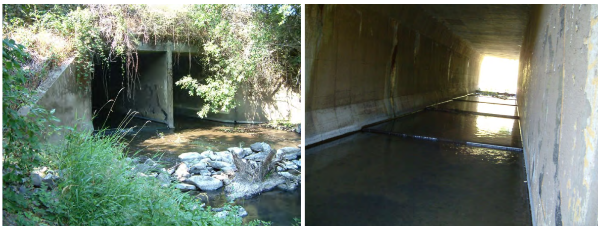
Figure 4.6: Site 04 – Oak Creek downstream and structure
