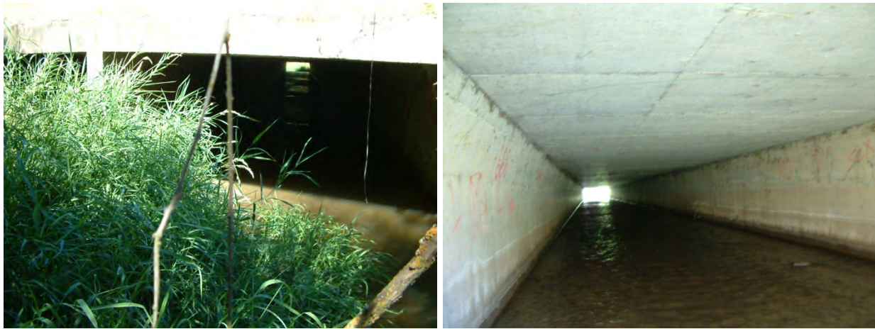
Figure 4.7: Site 06 – Griffin Creek downstream and structure
