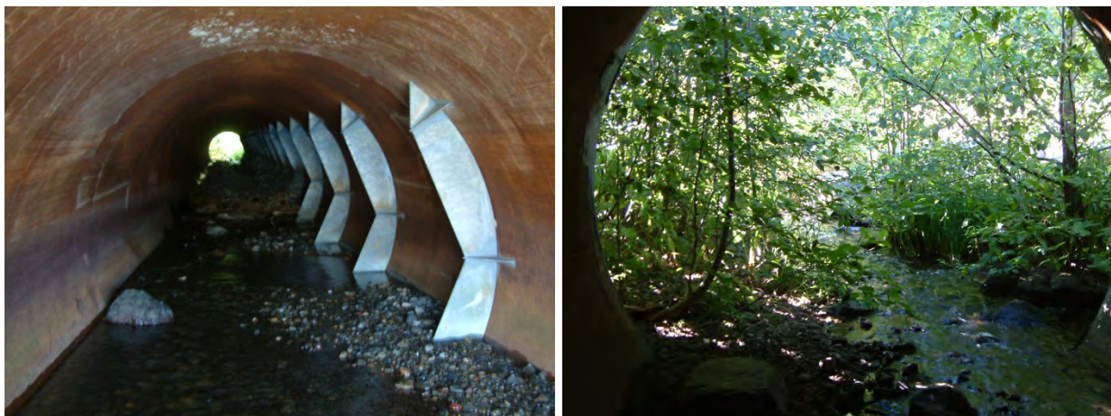
Figure 4.20: Site 18 - Perham Creek structure and upstream
