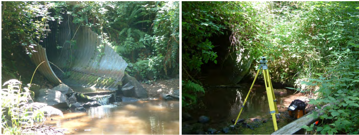
Figure 4.22: Site 20 - Tickle Creek downstream and upstream
