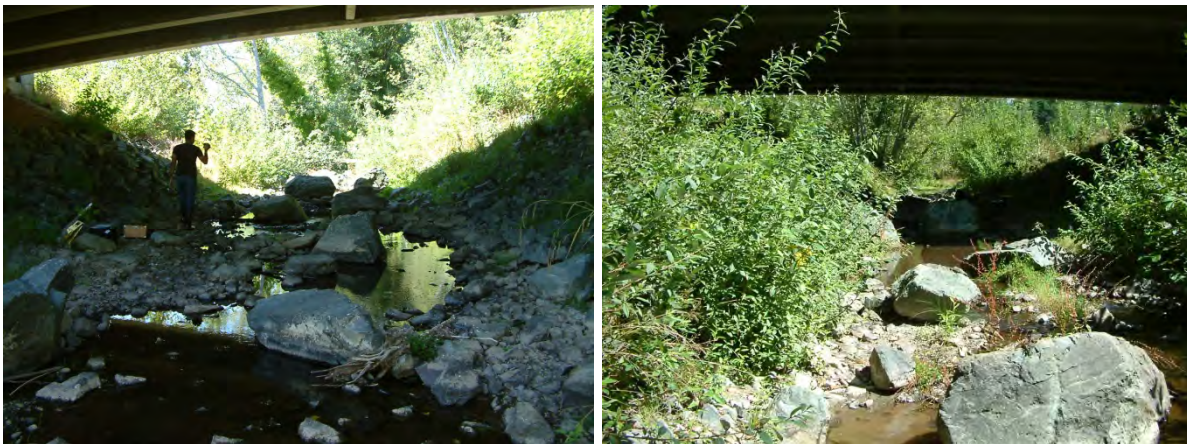
Figure 4.16: Site 14 - Bethel Creek under structure and downstream
