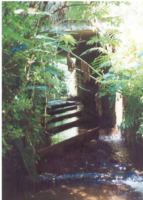
Figure 2.1: Example of Baffles in a Box Culvert
