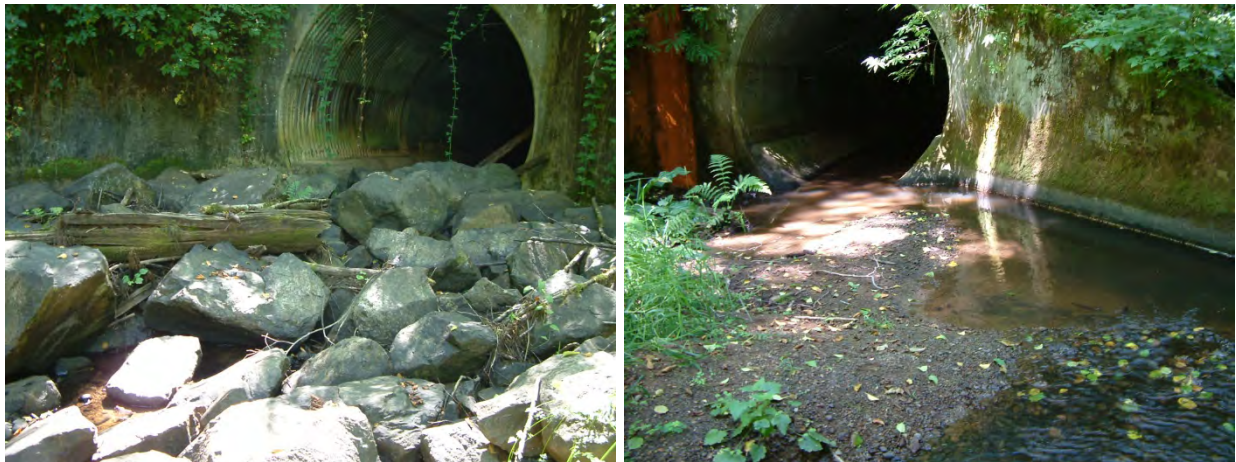
Figure 4.5: Site 02 – Mill Creek downstream and upstream
