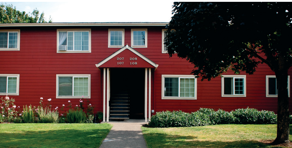
Elm Park Apartments in Forest Grove, Bienestar's first development built in 1984.
