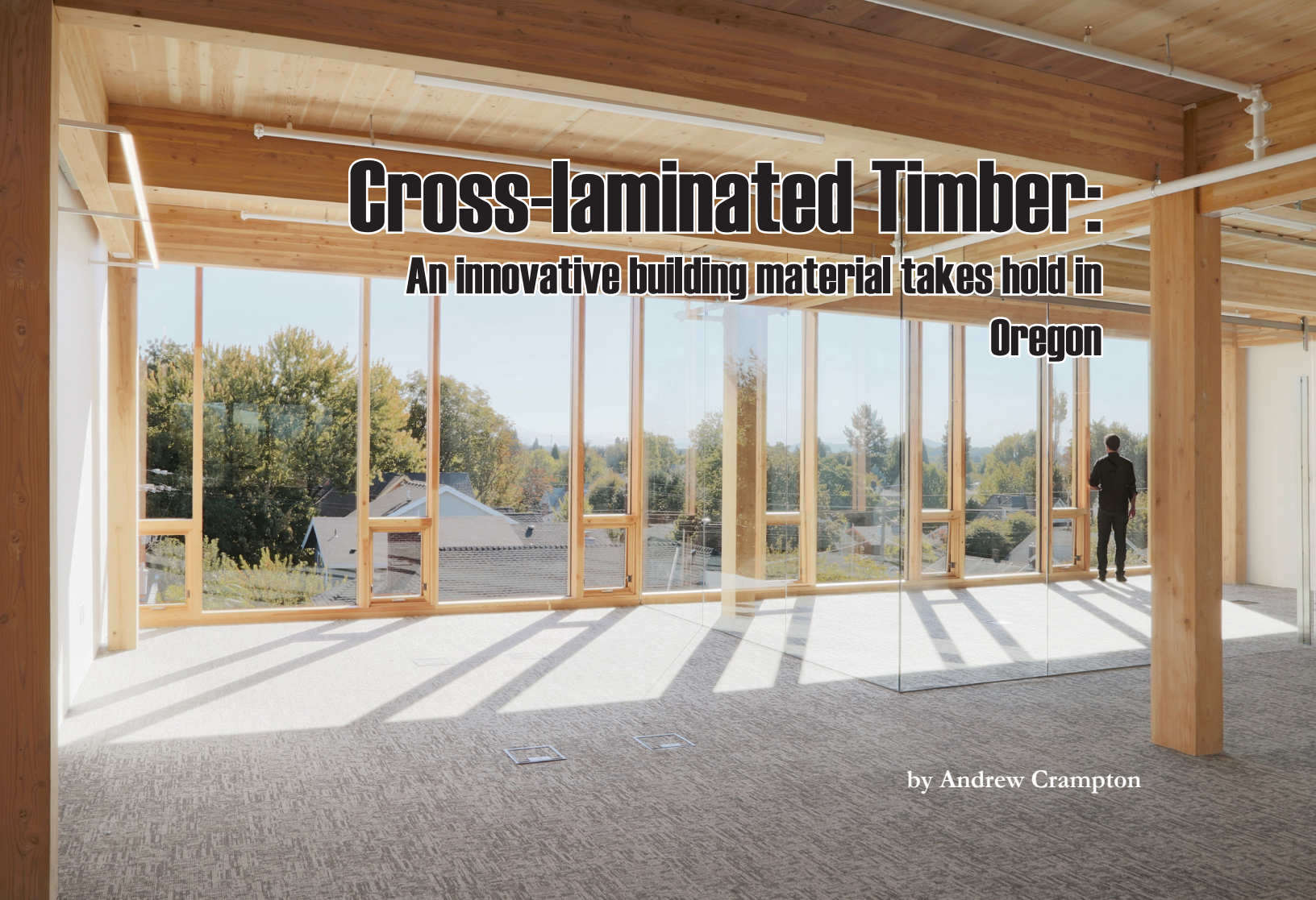
Figure 1: Albina Yard, a 16,000 sq. ft. creative office building currently under construction in North Portland's vibrant Mississippi District, is being constructed with CLT. Courtesy of LEVER Architecture
