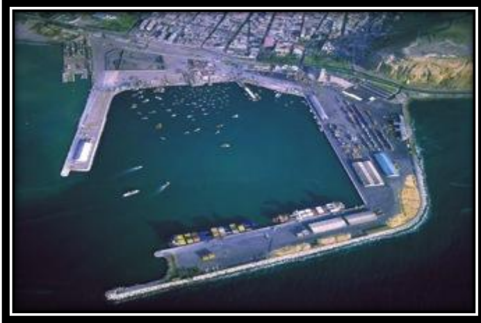
Figure 9: Port of Arica and "Irregular Triangle" 22
