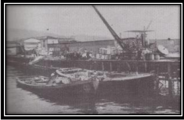
Figure 13: Photo of Barges and Cranes 39
