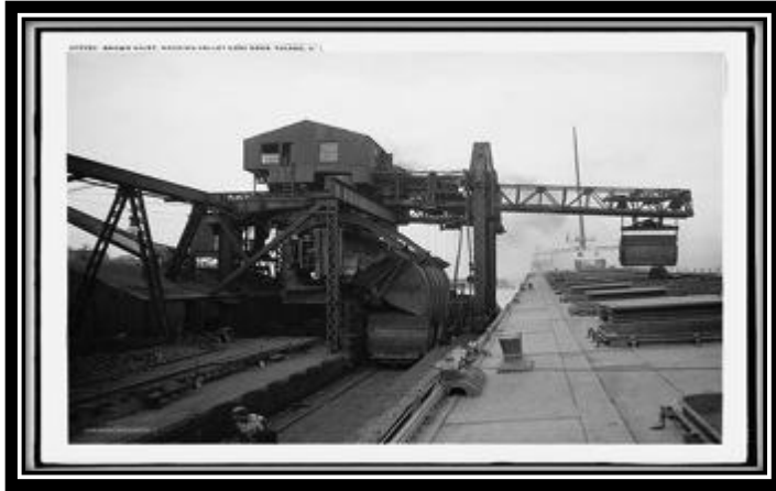
Figure 5: American Brown Hoist Crane 11
