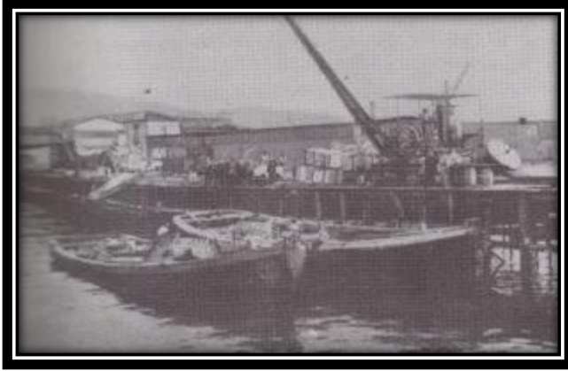
Figure 13: Photo of Barges and Cranes 39
