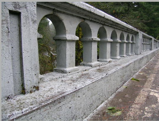
Gales Creek Bridge stonework. Photo by Michael Goff.
