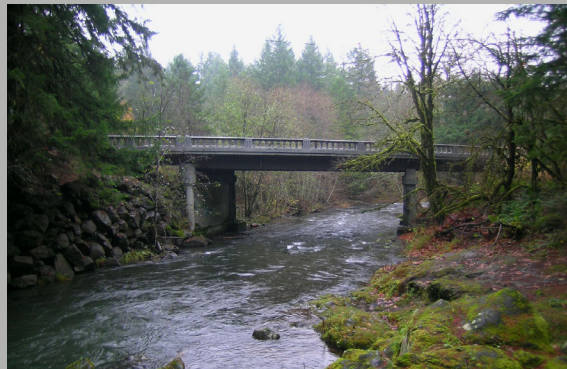
Gales Creek Bridge. Photo by Michael Goff.
