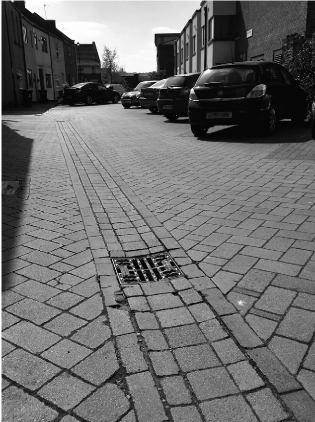
Figure 2. Permeable paving in the UK
