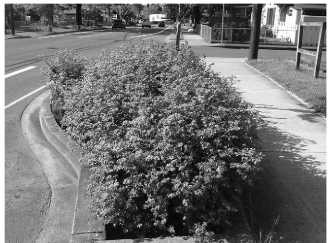
Figure 6. Bioswale with kerb-cut in the USA
