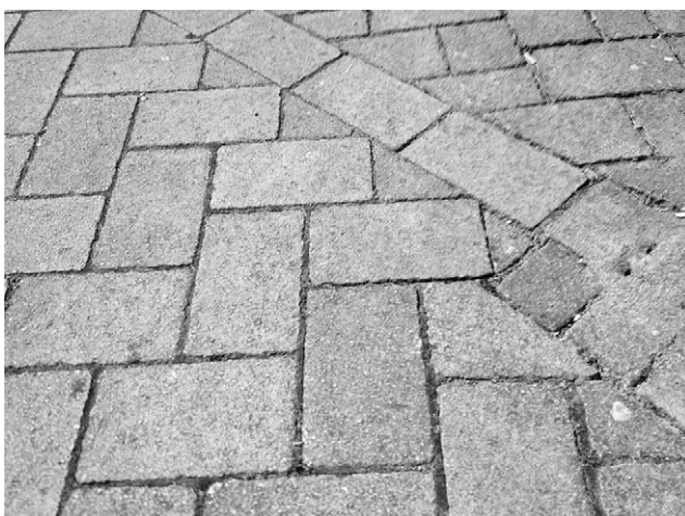
Figure 5. Permeable paving in the UK – close-up
