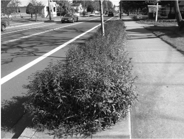
Figure 7. Bioswale without kerb-cut in the USA
