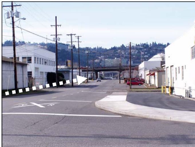
Looking down SE Division Place from the NE corner of SE 8th — a large turning radius for trucks increases the crossing distance to 64'. Pedestrians are encouraged to cross SE 8th on the south side.
