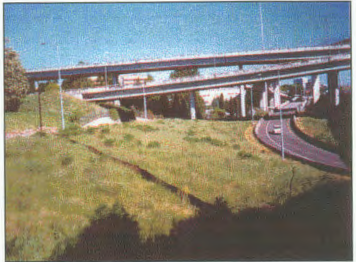
View of site, looking south
