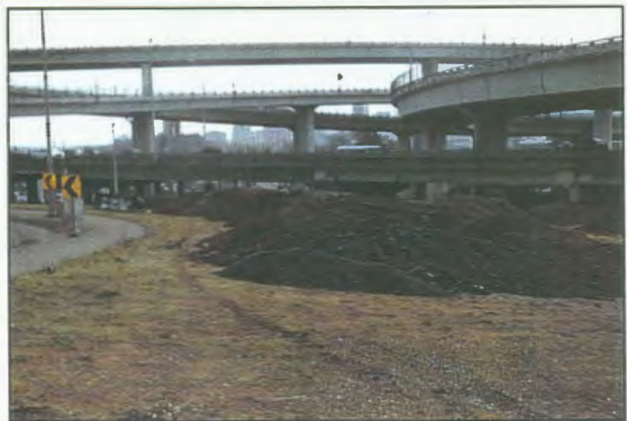
View of site, looking south
