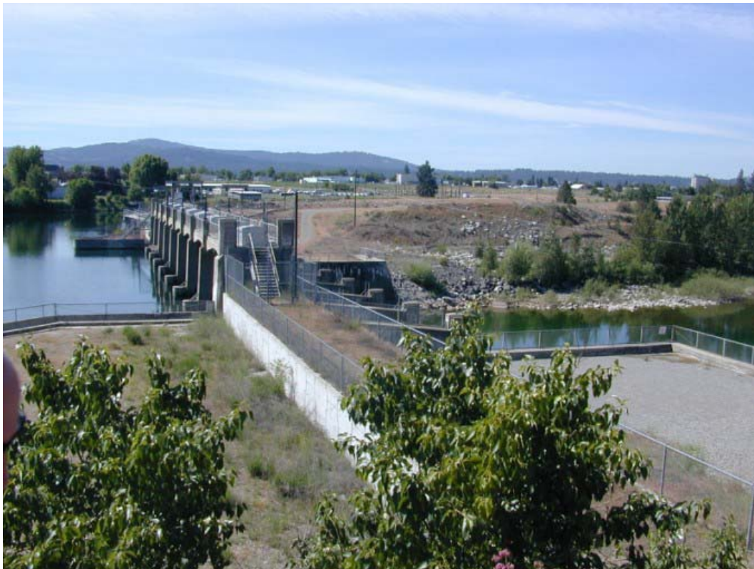
Figure 48. Upriver dam and spillway from North bank of the Spokane River
