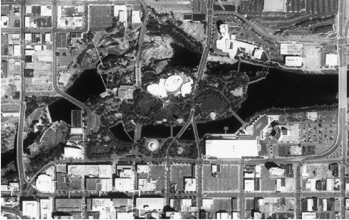
Figure 54. Upper Falls Dam and Monroe St. Dam in downtown Spokane, WA
