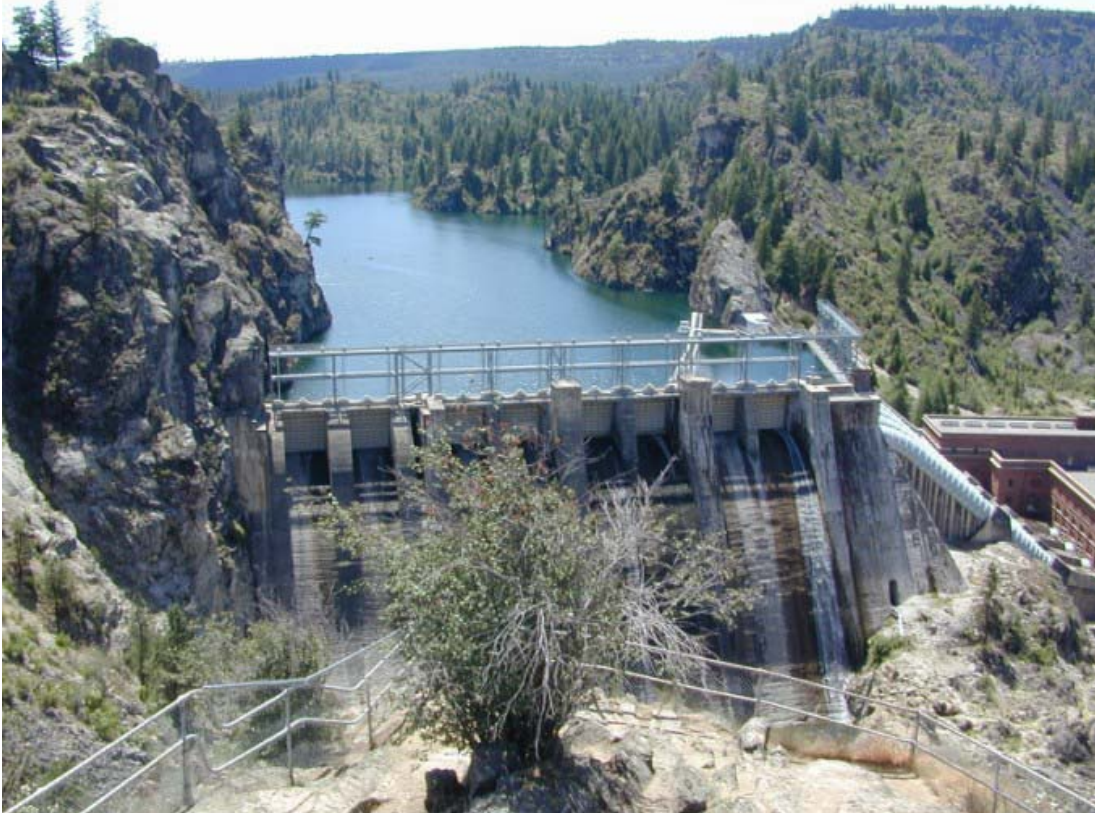
Figure 62. Long Lake Dam and Powerhouse
