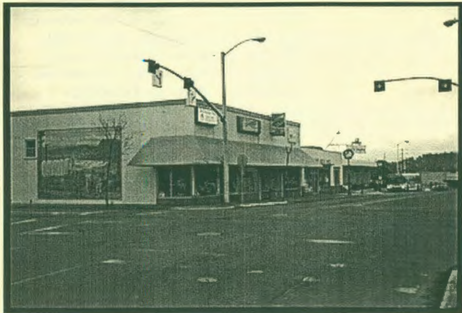
Looking north at the intersection of 10th Street and Main Street. Note the need for maintenance on the crosswalks. This intersection may also experience more traffic as a result of the opening of the End of the Oregon Trail Interpretive Center.
