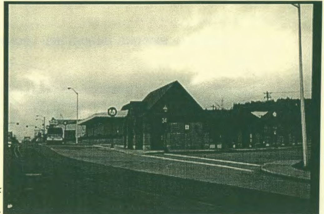
Tri-Met Transit Station at 11th Street. Note the lack of crosswalks for crossing Main Street.
