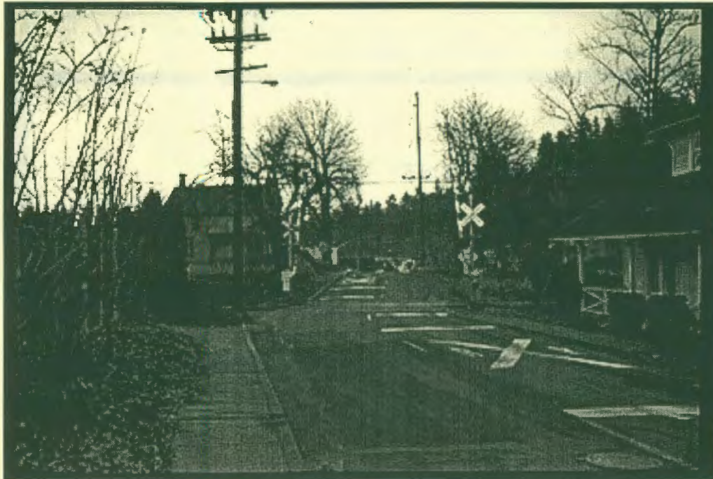
17th Street right-of-way facing east toward Washington Street. On the right side of the picture flows the Abernethy Creek. On the left is an electrical substation and after the tracks is the Hackett House. This area has incomplete sidewalks. High speed train traffic crosses 17th Street at grade. This area is not conducive to pedestrian traffic.
