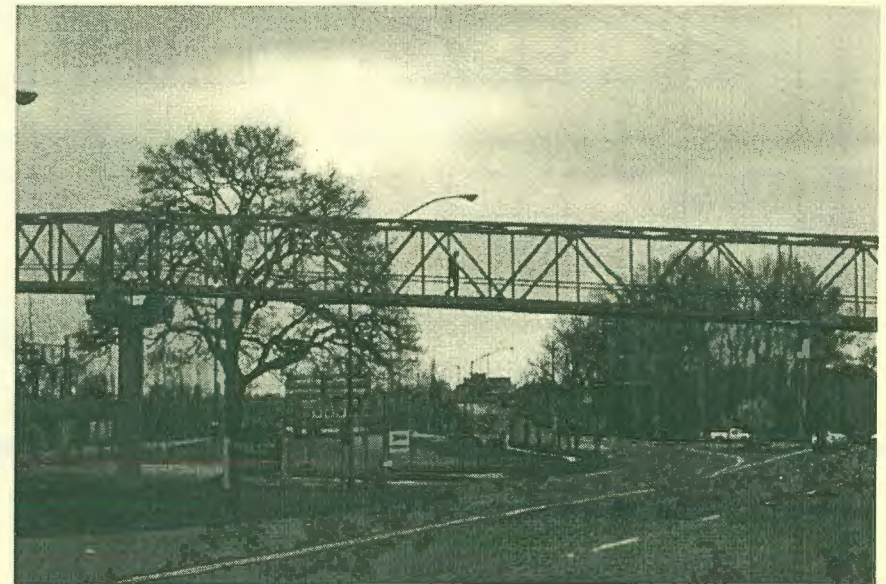
A pedestrian bridge located in Salem on the Willamette University Campus. This bridge crosses both 12th Street and the Southern Pacific Rail line.
