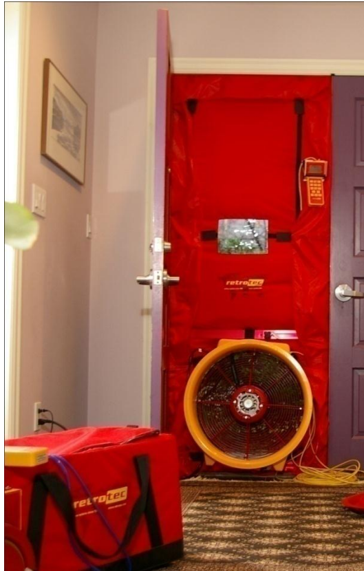
Figure 5: Blower door test photo
