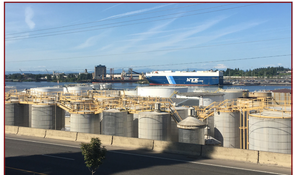
Figure 24: Petroleum Storage Tanks along NW St. Helens Rd.
