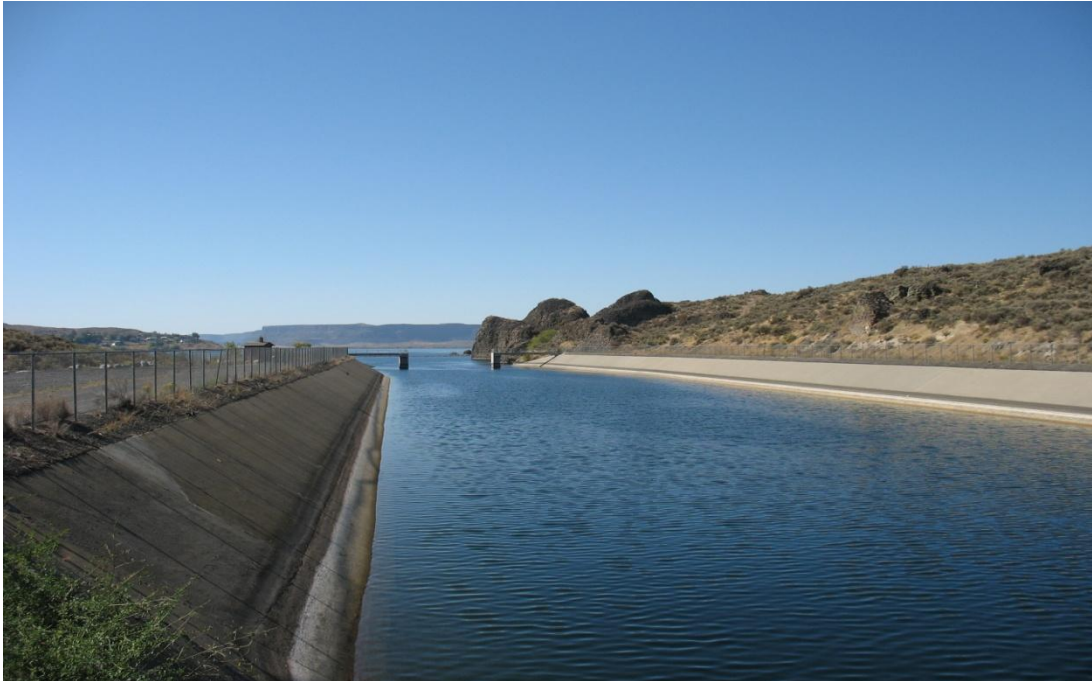
Figure 5. Banks Lake Feeder canal, facing South (Photo by Dr. Chris Berger)
