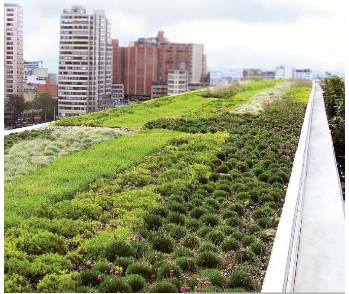
Figure 45. Example of Green Roof on Commercial Building
