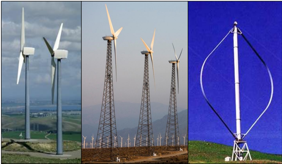
Figure M-1: Wind Turbine Tower Types
