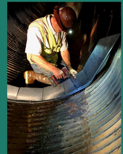
Above: Flexibaffles being installed at a culvert on North Fork Johnson Creek. These flexible baffles bend during high flows, slowing the velocity, and stay upright in low flows, creating resting pools.
