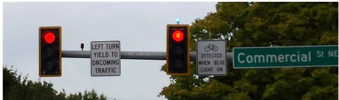
Blue Light and Explanatory Sign in Salem, OR (Source: ODOT)
