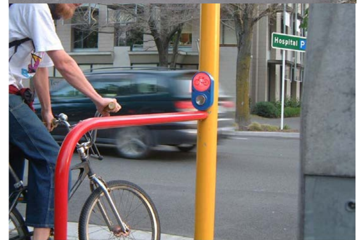
Nearside Confirmation System in Christchurch, NZ (Source: G. Koorey)
