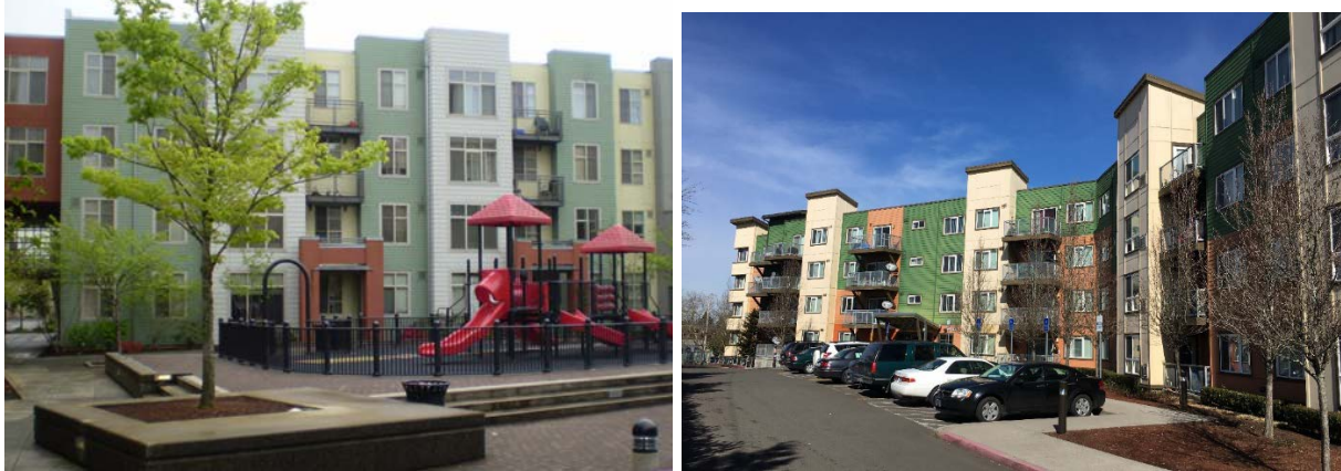
Figure 2-2 Center Commons (left) and Broadway Vantage (right)
