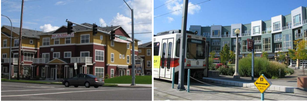
Figure 2-1 Elmonica Station Condominiums (left) and Beaverton Round (right)
