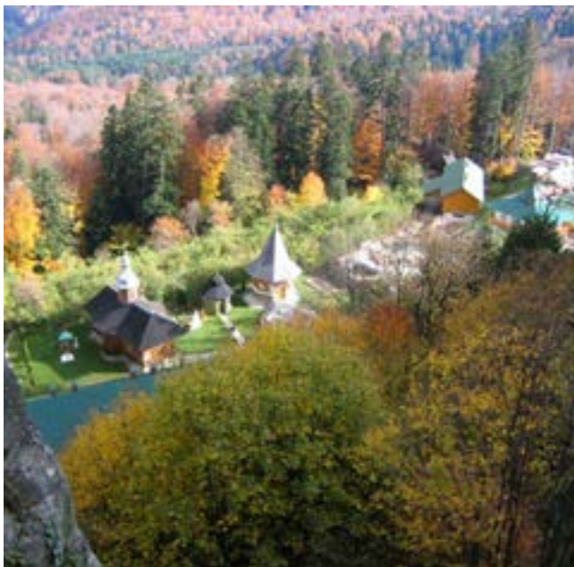
View of the new Skitul Sihla, under construction in 2007, from the ancient hermitage. © Josep-Maria Mallarach
