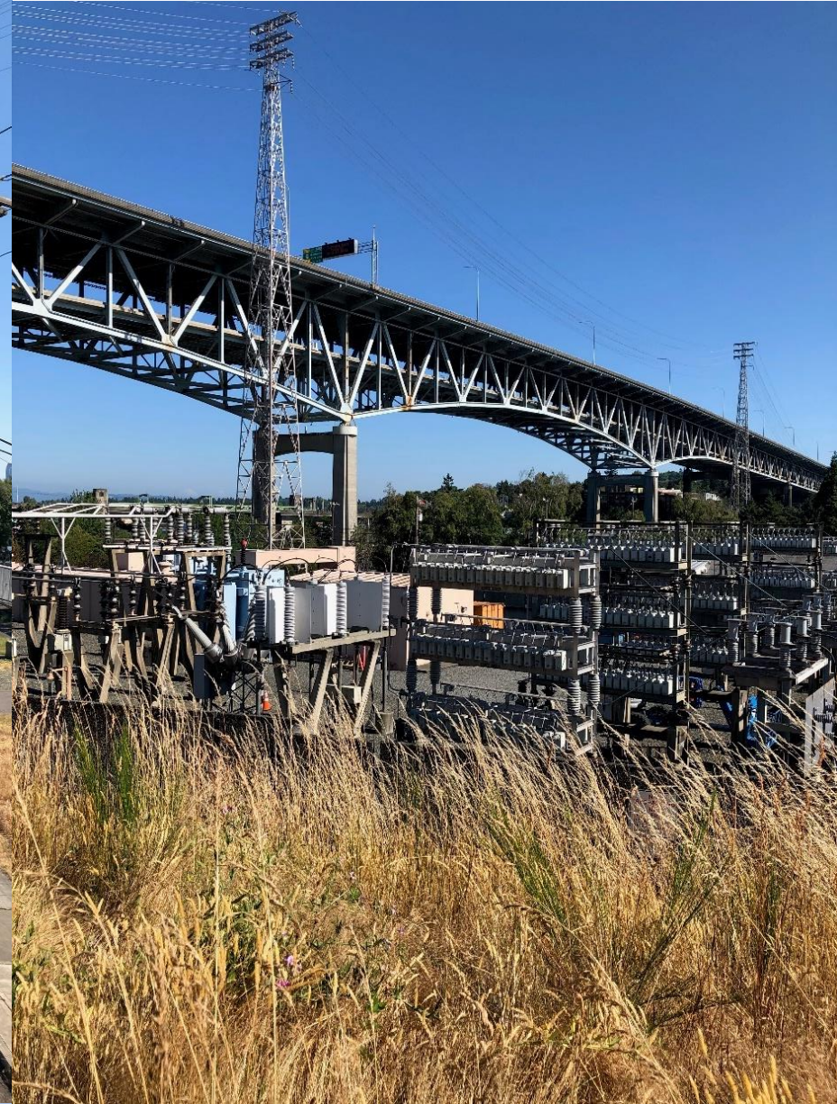
FIGURE 3.3 Interstate 5 over the Ship Canal in Seattle – huge and noisy structures attract industrial uses. Credit: Ralph Jenne
