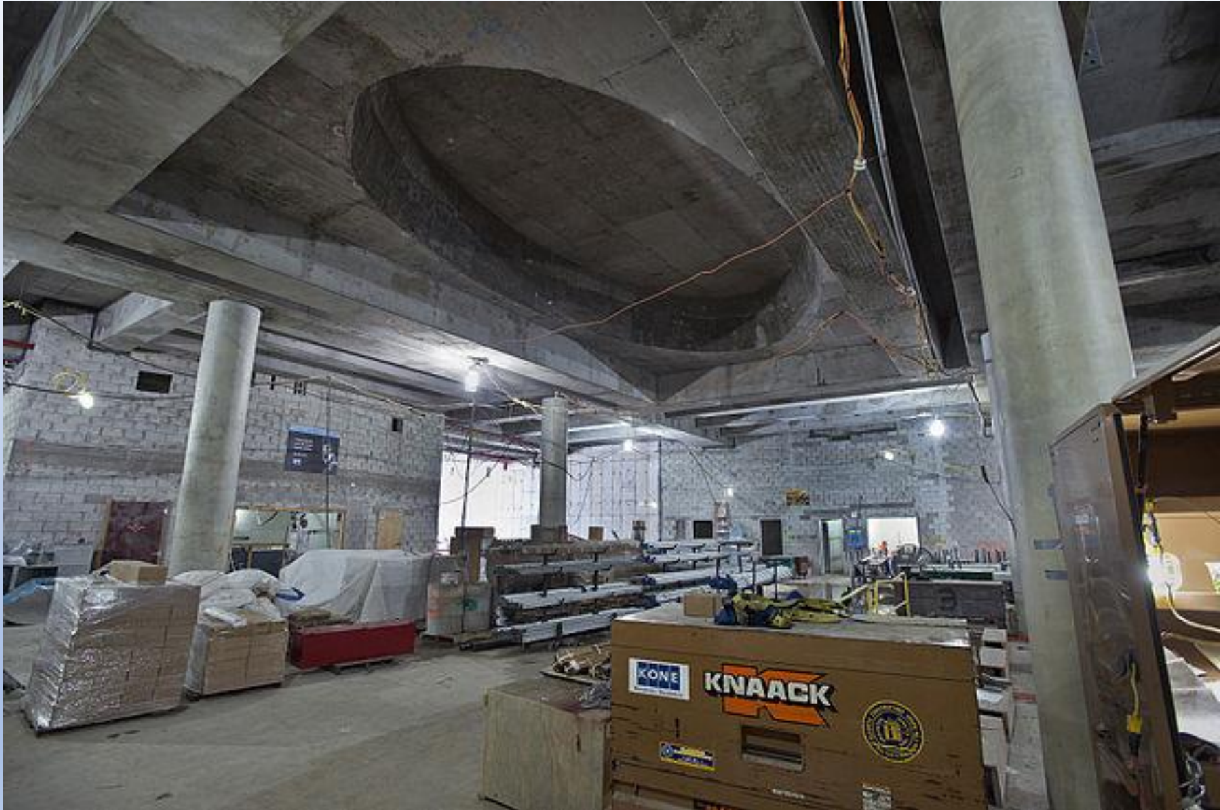
Figure 6.6 Hudson Yards (Jacob Javits Center) Station atrium under construction in 2013
