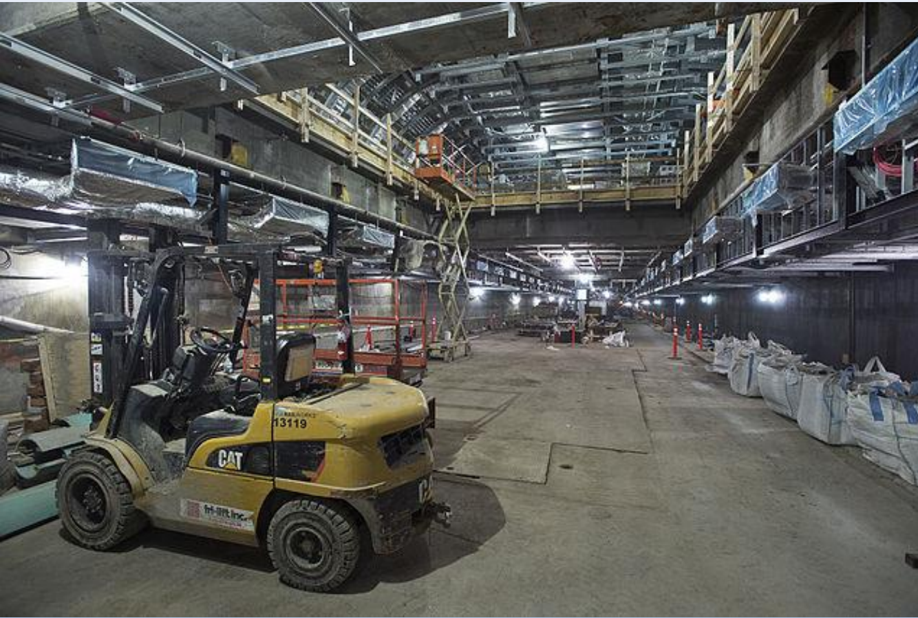
Figure 6.4 Size of station cavity for the line 7 extension at Hudson Yards (Jacob Javits Center) instead of more modest tube without mezzanines Credit : Metropolitan Transportation Authority / Patrick Cashin Creative Commons Attribution
