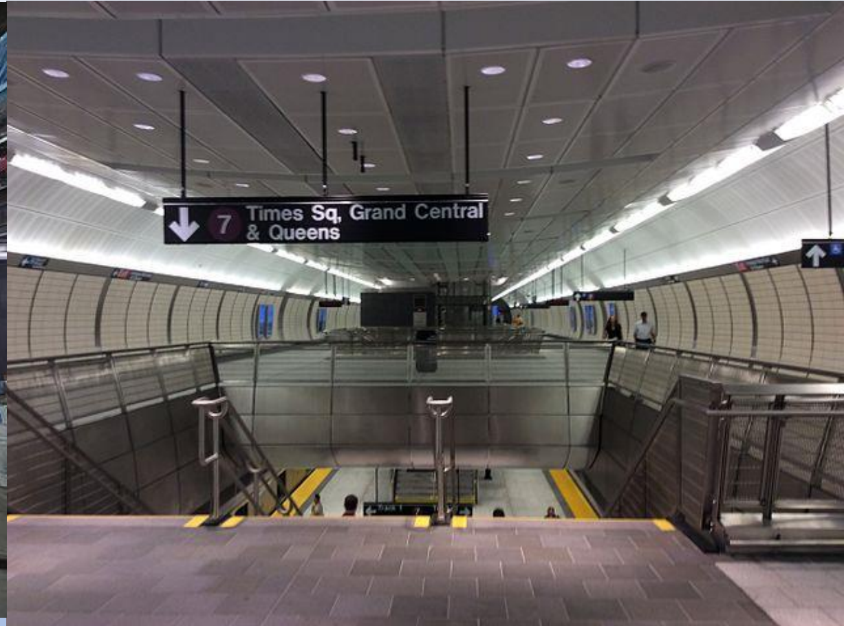
Figure 6.4 Size of station cavity for the line 7 extension at Hudson Yards (Jacob Javits Center) instead of more modest tube without mezzanines Credit : Metropolitan Transportation Authority / Patrick Cashin Creative Commons Attribution
