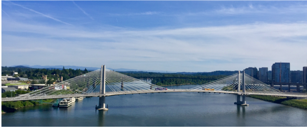
Figure 1.2: Tilikum Crossing spanning Willamette River looking south
