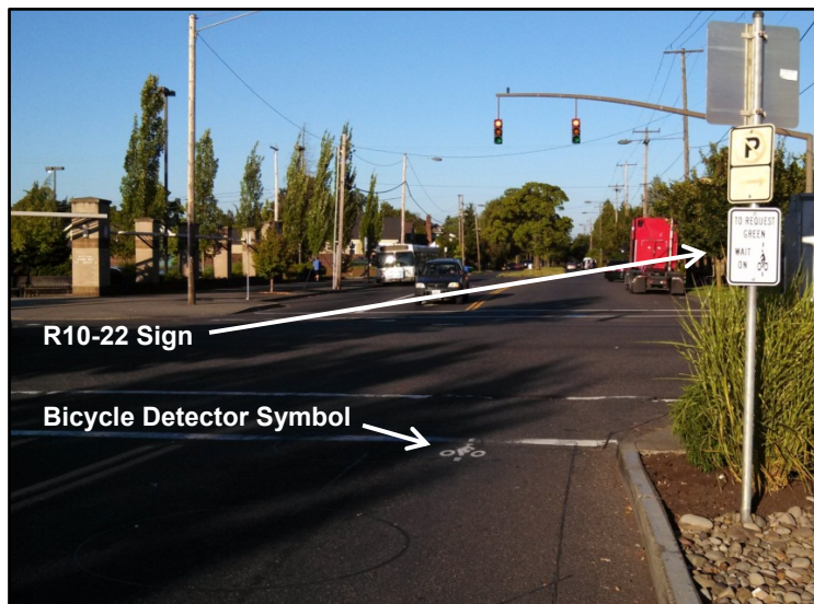
b) Site 2 After Modification – Bicycle Detector Symbol and R10-22 Sign
