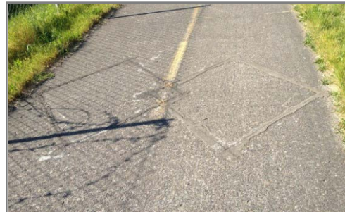
d. Double Diamond Bicycle Loop Detector on the I-205 Path at SE Yamhill St., Portland, OR
