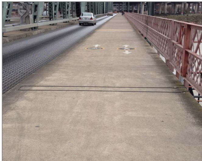
Figure 3.5. Permanent Pneumatic Tube Counter on the Hawthorne Bridge
