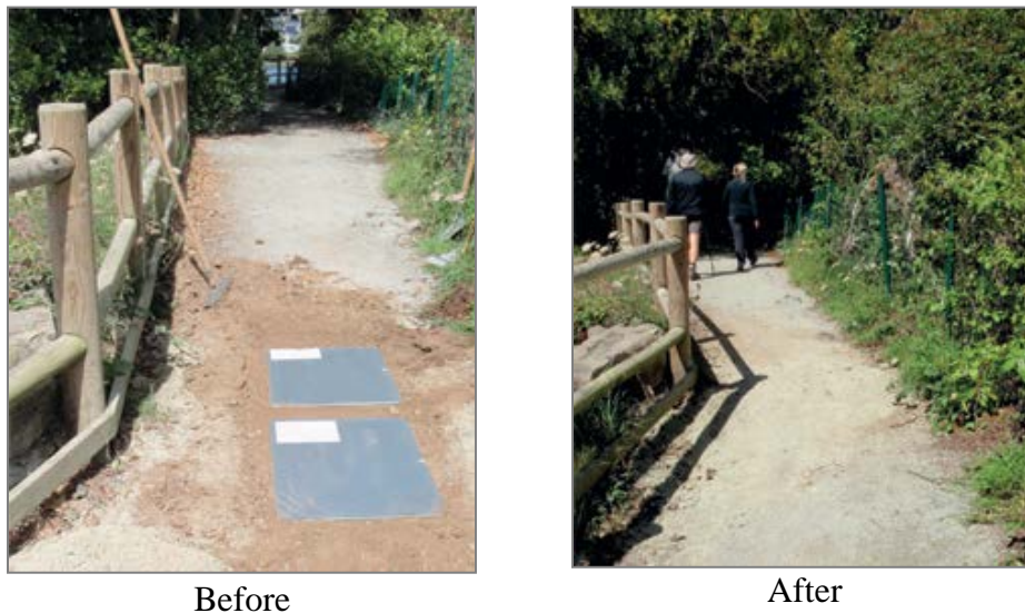
Figure 3.12. Installation of the EcoCounter Acoustic SLAB ( EcoCounter 2013 )
