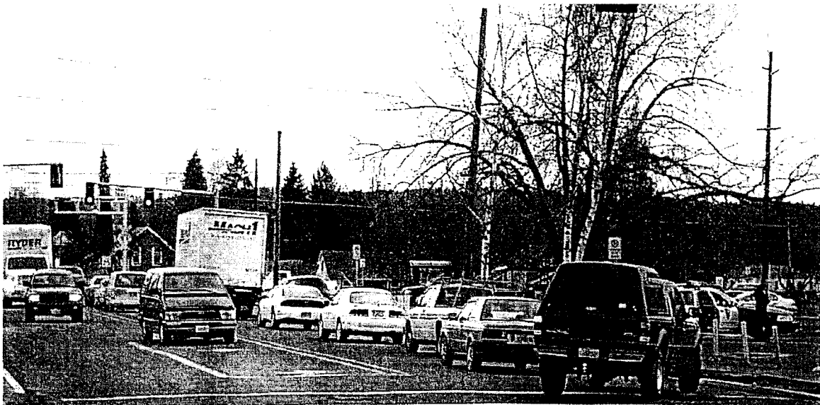
Standing at NE corner of TV Hwy (N Adair Street) & N 10th Avenue, looking south. Note traffic stacking from signal at Baseline Street, which sometimes results in partial blockage of N Adair Street's left travel lane.
