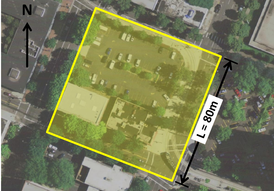
Figure 27: Representative unit chosen for estimating heat from vehicles. 4 th Avenue is the three lane, one-way street running southwest to northeast on the right side of the figure. Harrison Street is the two lane, two way street running along the bottom. The traffic counter is placed on 4 th Avenue one block northeast of the highlighted area. The unit is taken to be square, so A = L^2 = 6400 \text{ m}^2 . Image courtesy of City of Portland.
