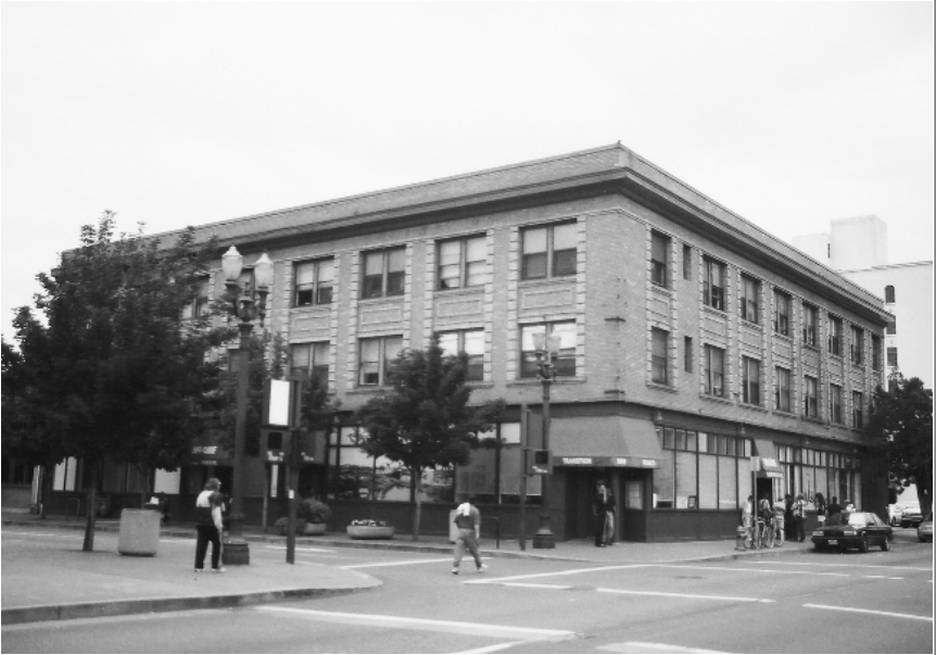
Figure #5: Transition Project, Inc. Men's Shelter
