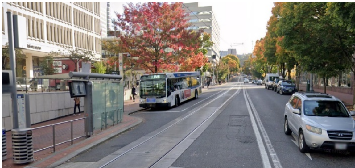
15 Figure 4 Transit mall: bus stop, bus bay, and sightlines of upstream light rail cars (Google Earth) 16 17
