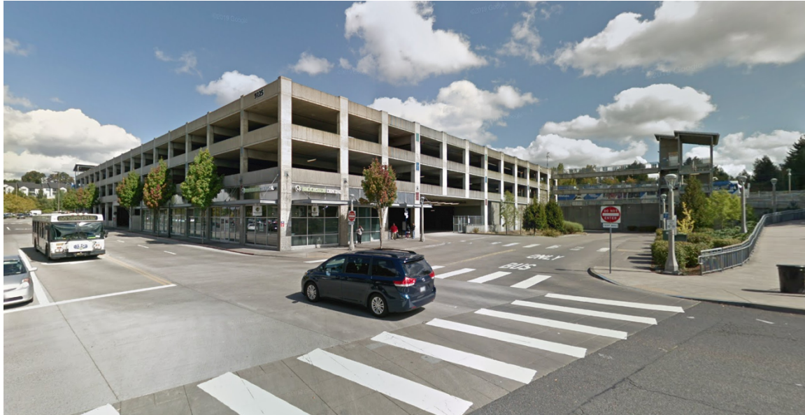
1 2 Figure 3 Street view of the Clackamas TC covered parking facility (Google Earth) 3
