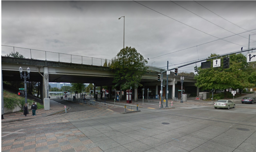
7 8 Figure 5 Street view of light rail stations at the Rose Quarter TC 9
