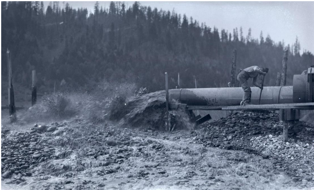
Debris from Willamette Heights filling Guild's Lake, April 21, 1924. Oregon Historical Society Research Library, bb006685
