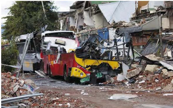
Many brick buildings collapsed and caused considerable damage around them during the 2011 magnitude 6.3 earthquake in Christchurch, New Zealand.
