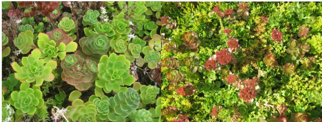
Photo 6: Close up of sedum foliage coverage with no visible soil exposure.
