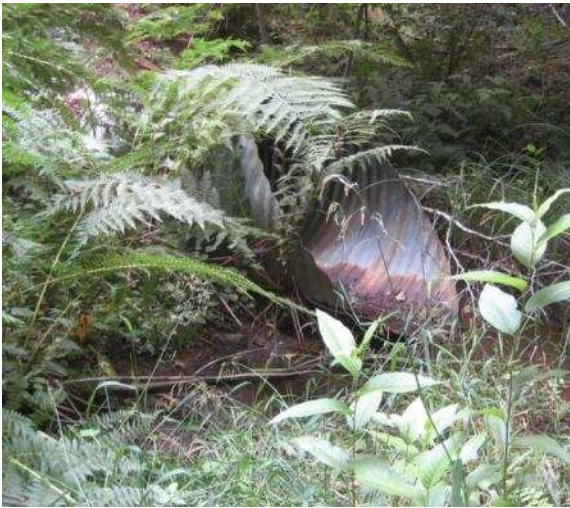
Site 2B Culvert
