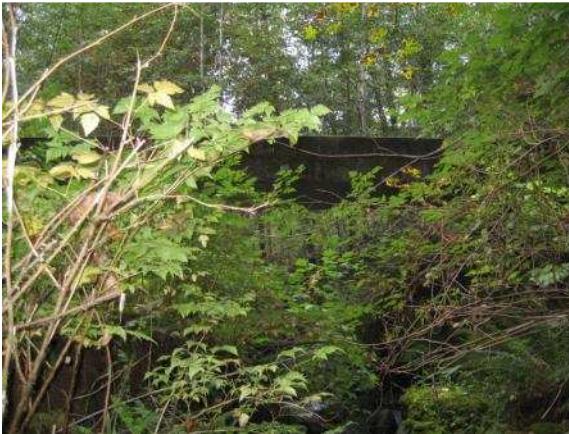
Site 11B Looking Downstream
