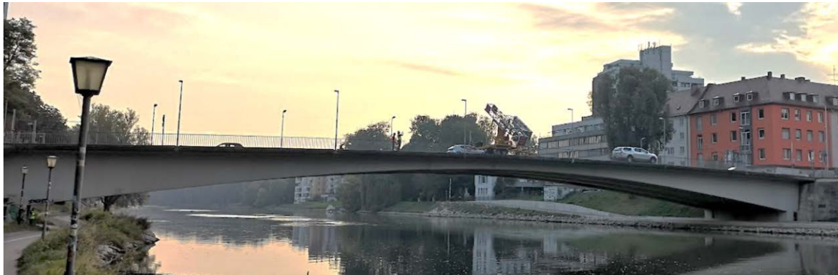
Figure 3: Photo of Gänstorbrücke, built 1950, prestressed concrete, over the river Danube from Ulm to Neu-Ulm. Some tendon wires suffer from 50% cross section loss due to corrosion [2].
