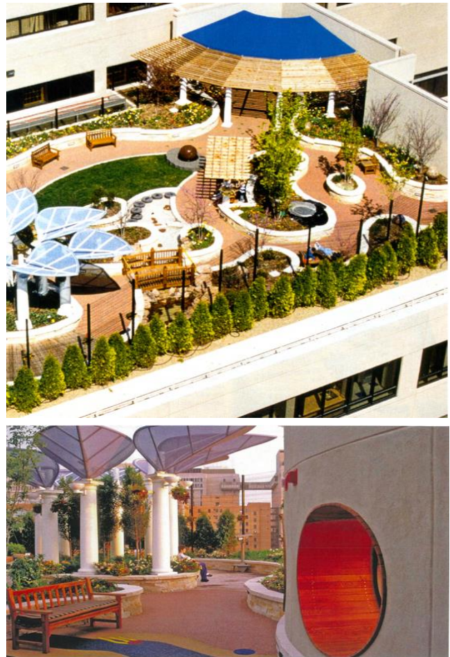
Figure 4: Photos of an accessible green roof in the Olson Family Garden at St. Louis Children's Hospital.
