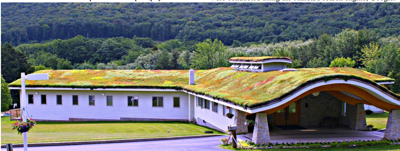
Figure 1: Photo of green roof at the Life Expression Wellness Center in Pennsylvania provided by study participant.
