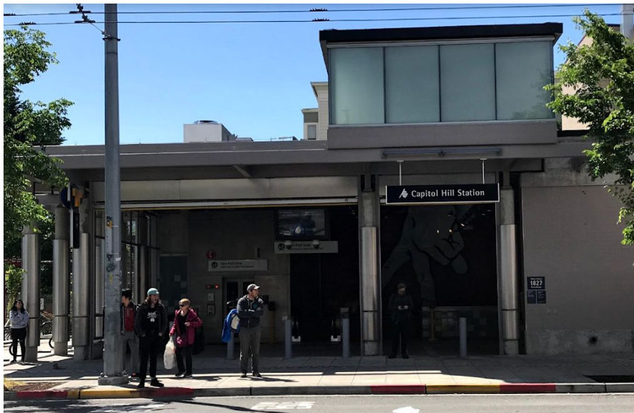
Image 10: Capitol Hill Station entrance. Photo by Antonio Crosier.
