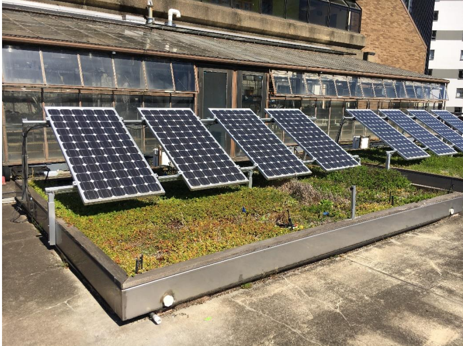
Figure 3. Experimental ecoroof platform on the SRTC rooftop (Facing Northeast).
