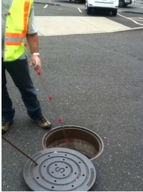
Figure 5: Todd Gunter, of the BES, collecting stormwater solids from sedimentation manhole using the described piping system
