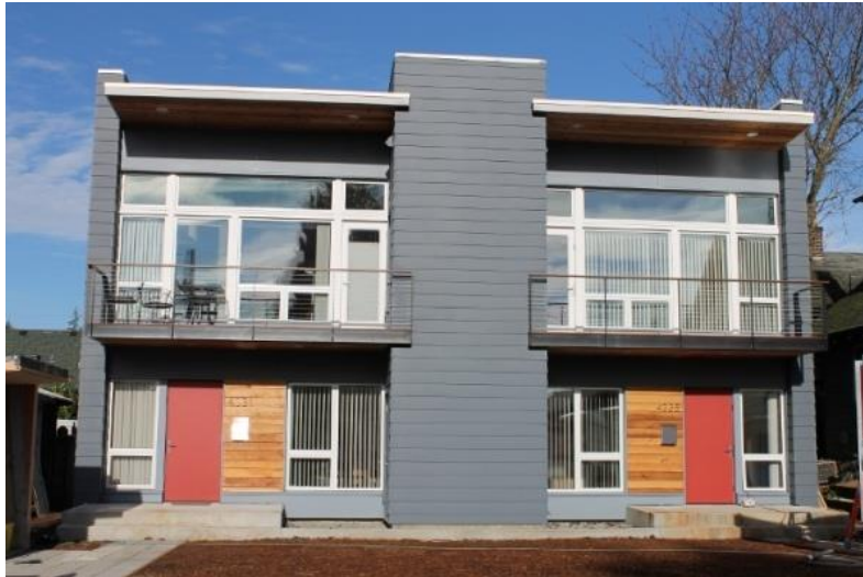
Figure 2.2. Trekhaus, a passive house duplex home, is divided into two mirror-image apartments with a party wall on the north-south axis.
